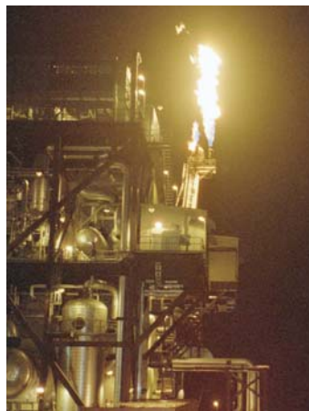
Natural gas flare
